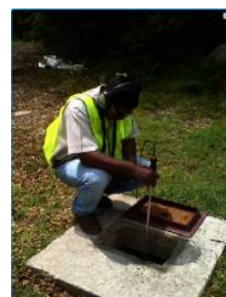
Fig.9 listening directly on a Valve or Hydrant
